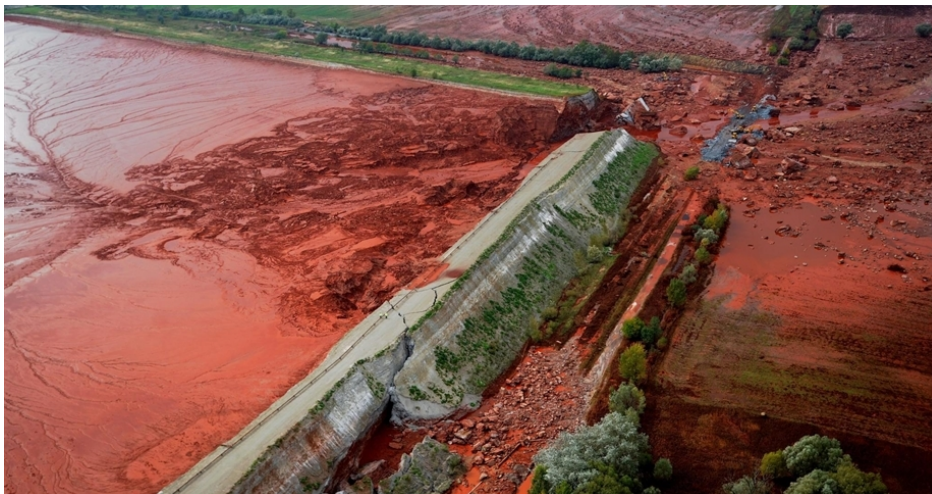
Figure 1.: The damaged dam of the reservoir
